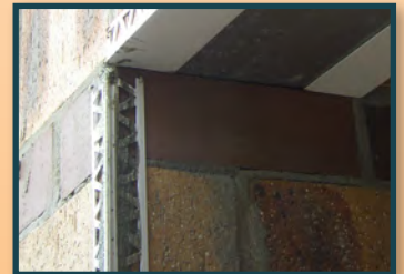
The perfect bond - the patch render and render finish will blend together
